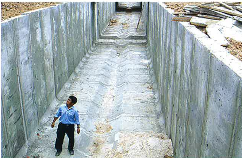
R.C. Open Drains with DWF Section
