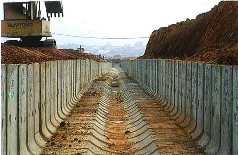
R.C. Open Drains with DWF Section
