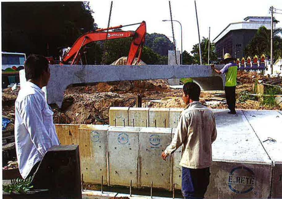
Installing Segmented Box Culverts
