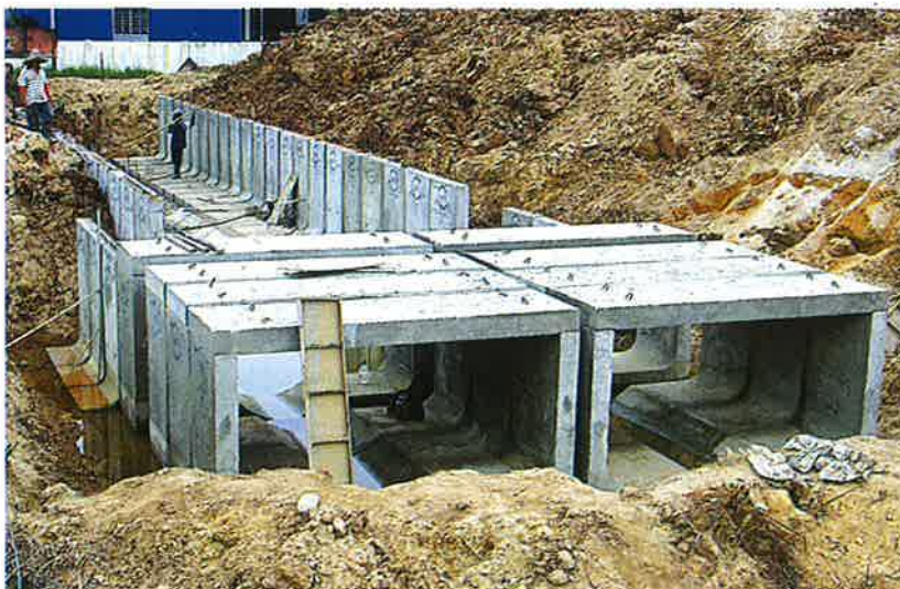
R.C. twin Large Box Culverts & 'L' Shape Unit.
