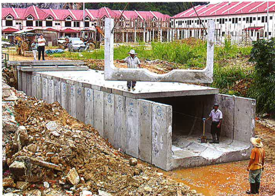
Installing R.C. Large Box Culverts
